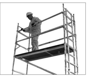
Dismantling is the reverse except when dismantling the handrail braces. Unclip the far end hooks and then from the sitting position through the trapdoor (3T) remove the handrails. Do not remove the handrails whilst standing on the platform, this would leave you at risk.
