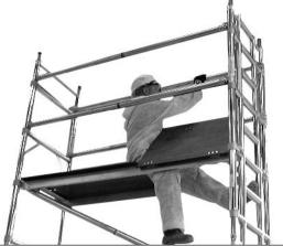
From the sitting position through the trapdoor (3T) 12 fit four handrail and mid rail braces to the vertical members.
