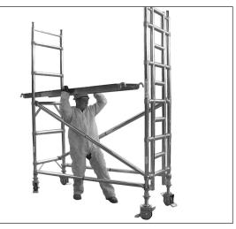
5 Fit trapdoor platform on appropriate rung, see tower illustration for guide. This will indicate which rung to fit trapdoor platform depending on final height.
