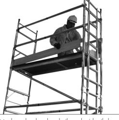
Fit toeboards when handrails and mid rails have 13 been correctly fitted. For intermediate work, platforms, handrails, mid rails and toeboards must be fitted
