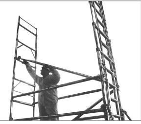
Klik in diagonal braces to continue in a regular pattern from rung to rung except when interrupted by an intermediate trapdoor platform.
