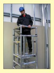
Horizontal braces complete the guard rail around the top working area.
